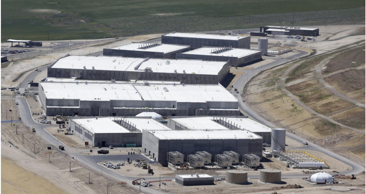
UTAH Data storage center
