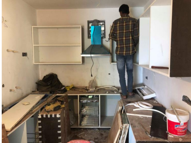
Working on the kitchen.
