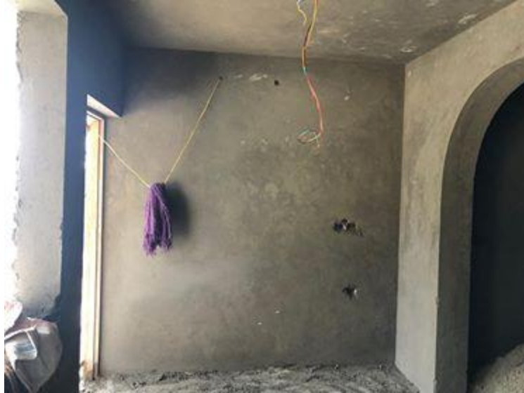
Inside the downstairs
