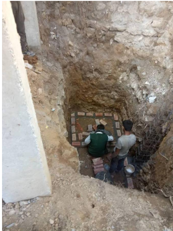
Putting in the sewage.
