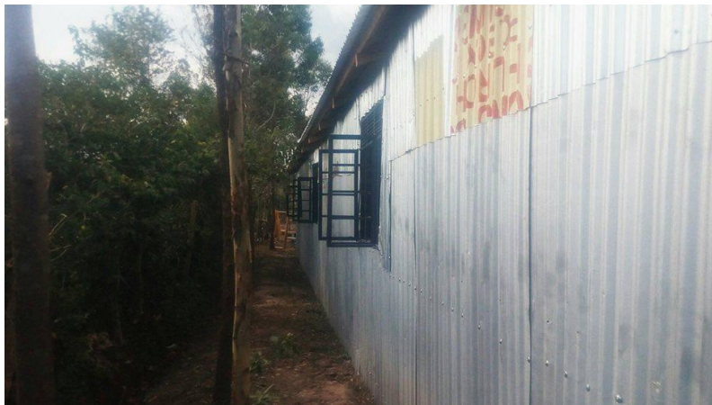
The windows are in
