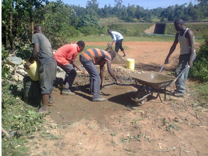
Working on the foundation for the toilets.
