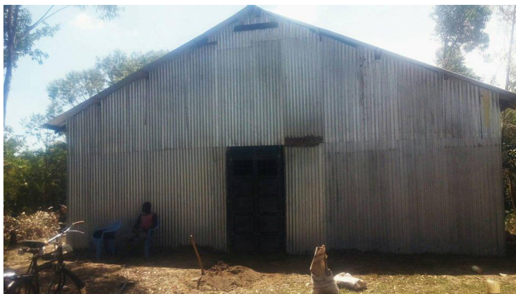
Here is the front.
