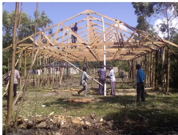
The church building is going up!
