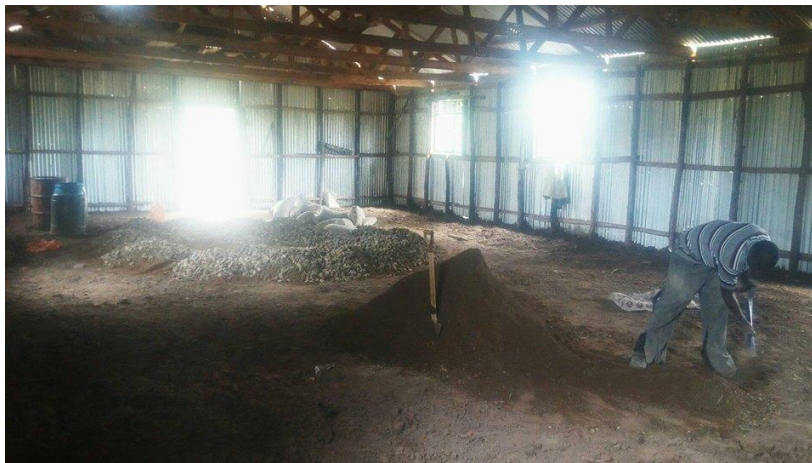
Beginning the work on the floor
