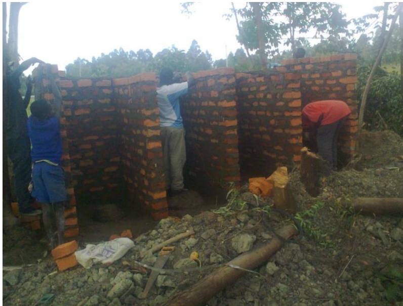
Walls going up
