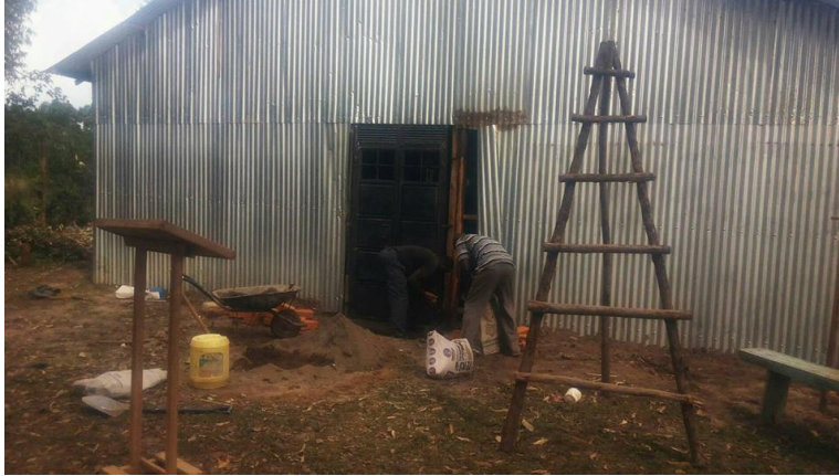
Working on the front of the church
