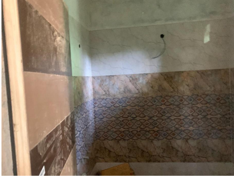
This is showing the pretty tile work in the bathroom.
