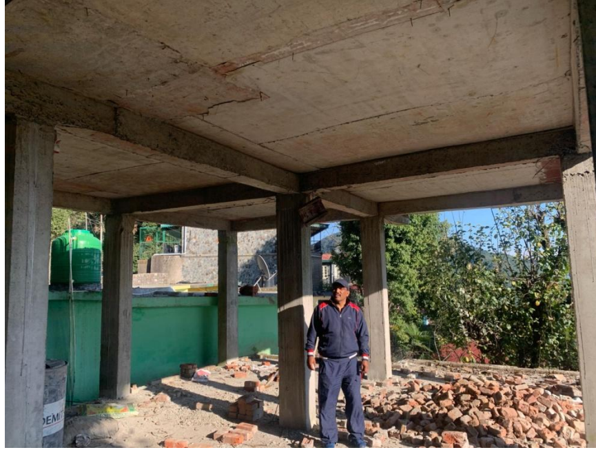
Upstairs where the church will be.
