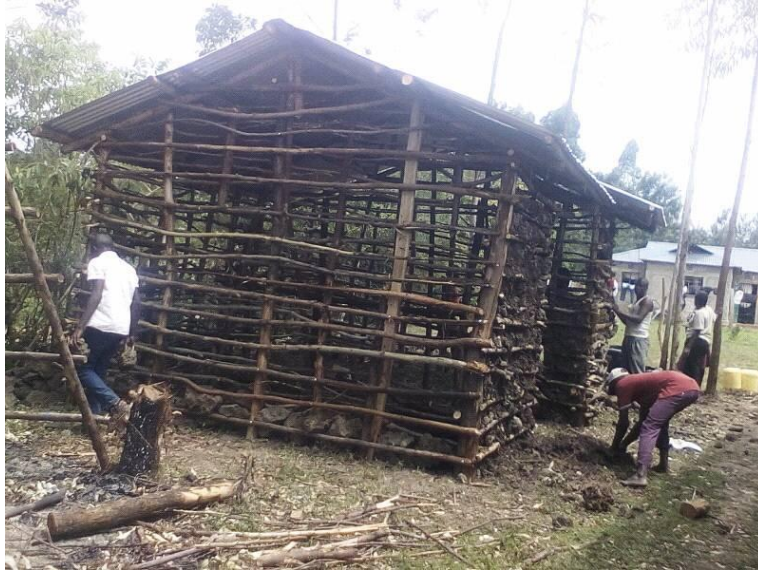
Here they are working on the kitchen
