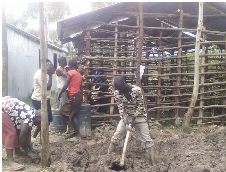
Getting the dirt ready to be mud for the walls.
