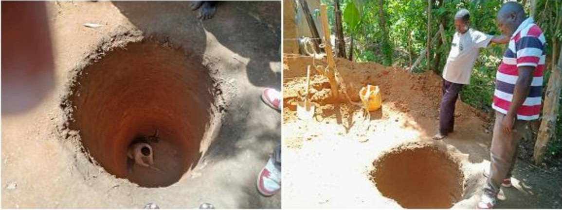
Picture of the water well being dug
