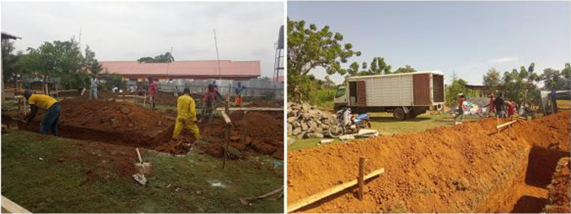
Starting to dig the foundation.
