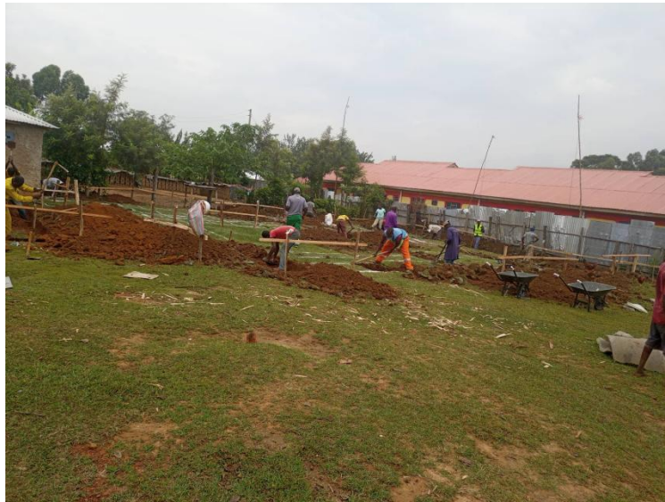
Working on the form.
