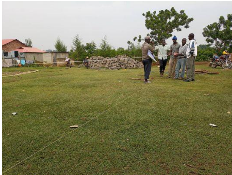
Beginning to lay the lines for the foundation of the house.
