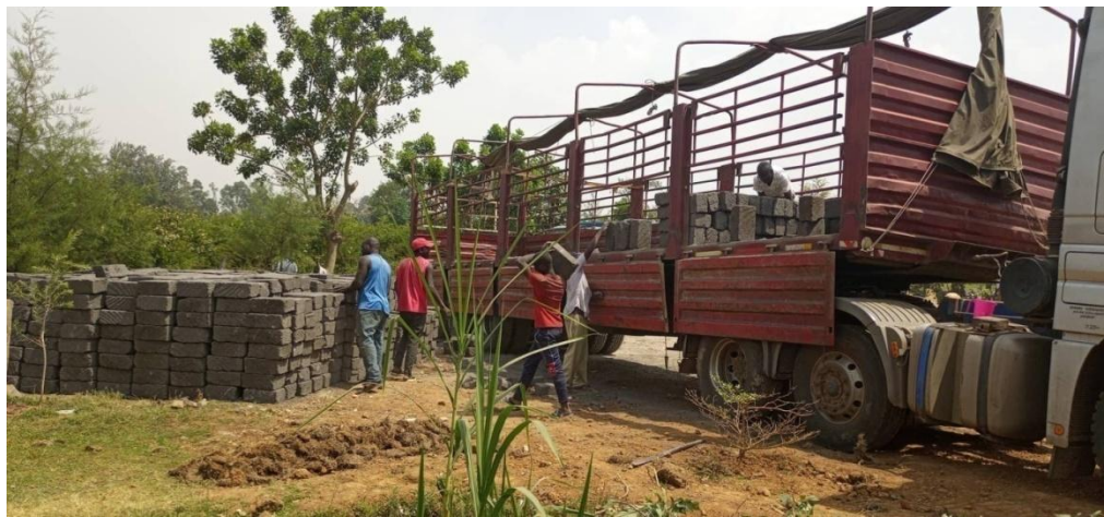
They are unloading some kind of cement blocks.
