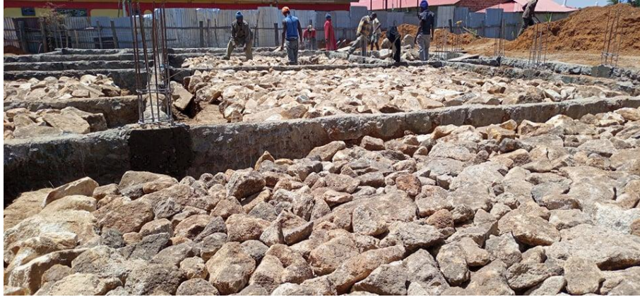
Filling the foundation with rocks and dirt.
