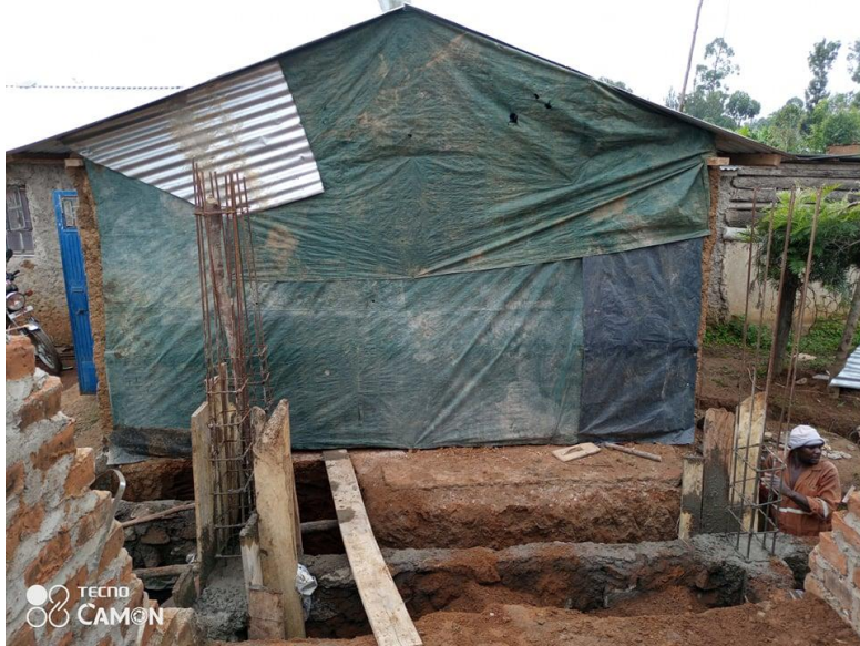
Here is a better picture of no living room, they have placed a tarp to close of his home. He's been living without a living room for many months now.
