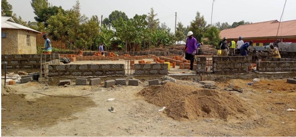
Here are the ground floor walls going up.
