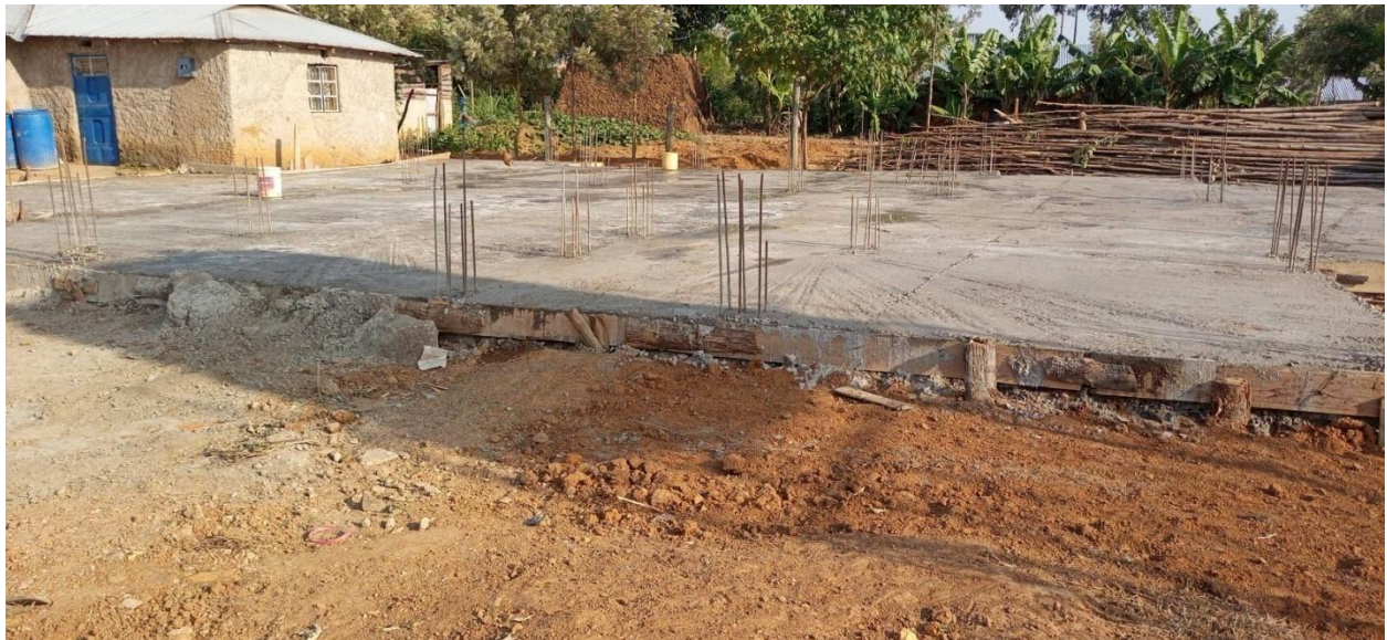
Filling the foundation with rocks and dirt.
