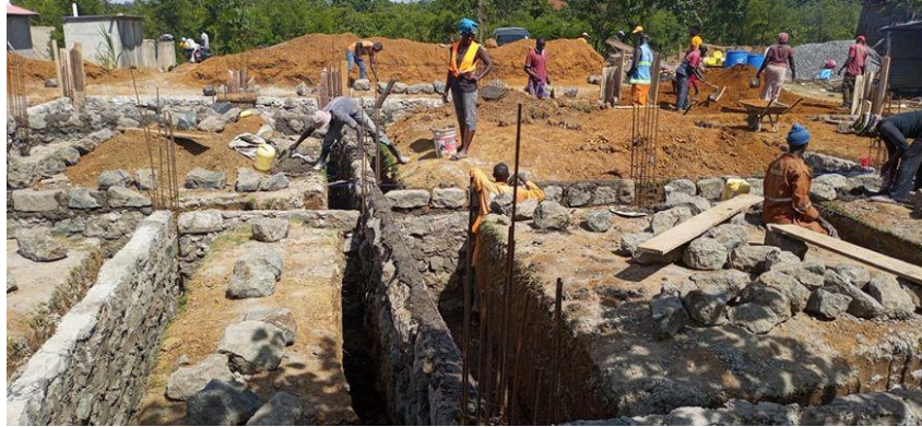
Working on the foundation.
