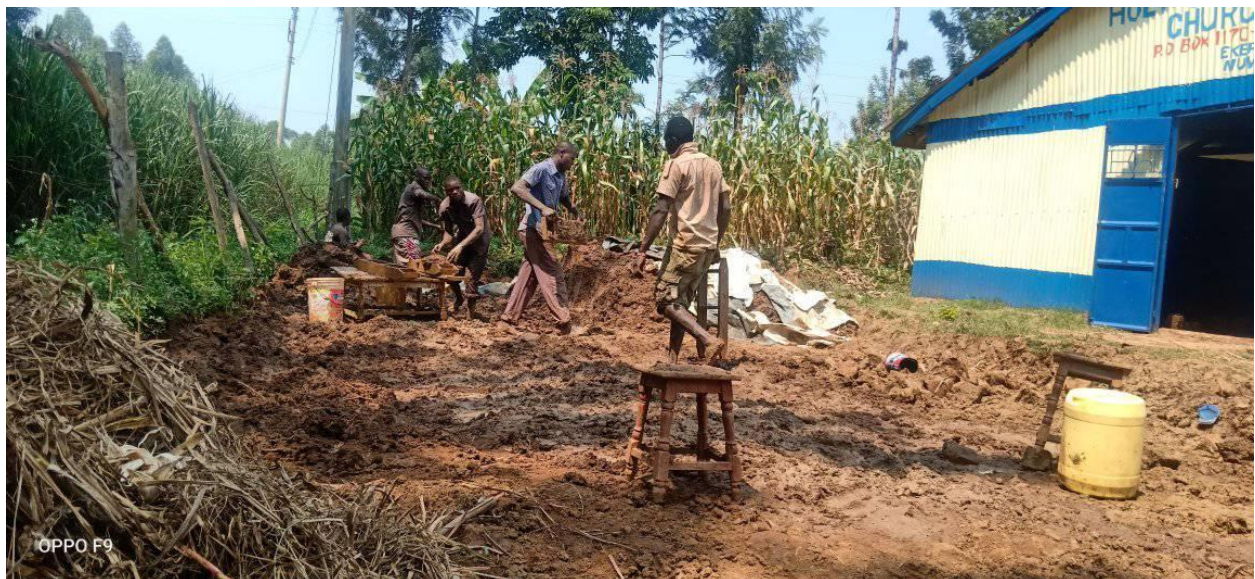
Still doing the work.
