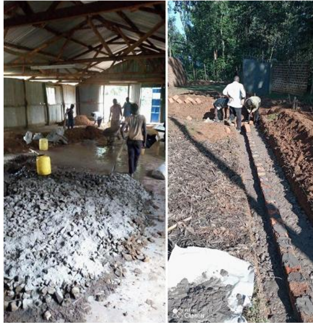
On the left they are making a concrete floor for the church and on the right they are beginning to lay the foundation of bricks for a wall of the church.
