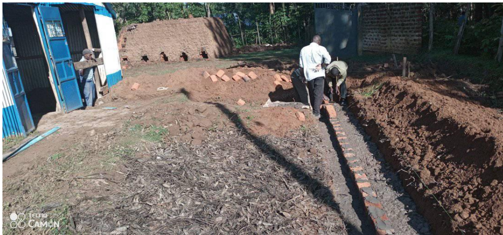
On the left they are making a concrete floor for the church and on the right they are beginning to lay the foundation of bricks for a wall of the church.
