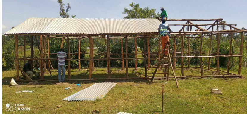
The roof is being put on.
