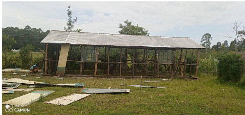
Now they are starting to work on the sides.
