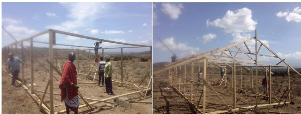
The church construction is underway.
